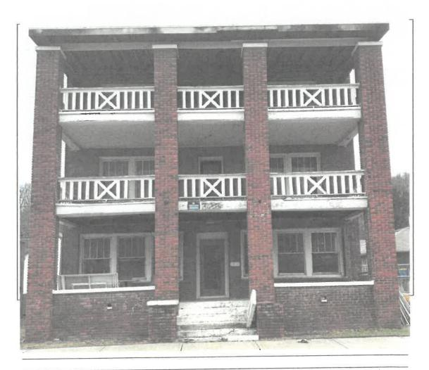
Outer patios will be rebuilt. They will be rebuilt in the same historic manner. The railing will be raised to provide the required height. The windows will be painted white to match the currnet color.
