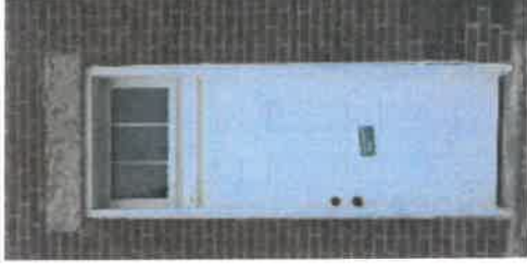
Example of inappropriate door replacement. The replacement door is too short and does not fit into the door opening. (STRATA)
