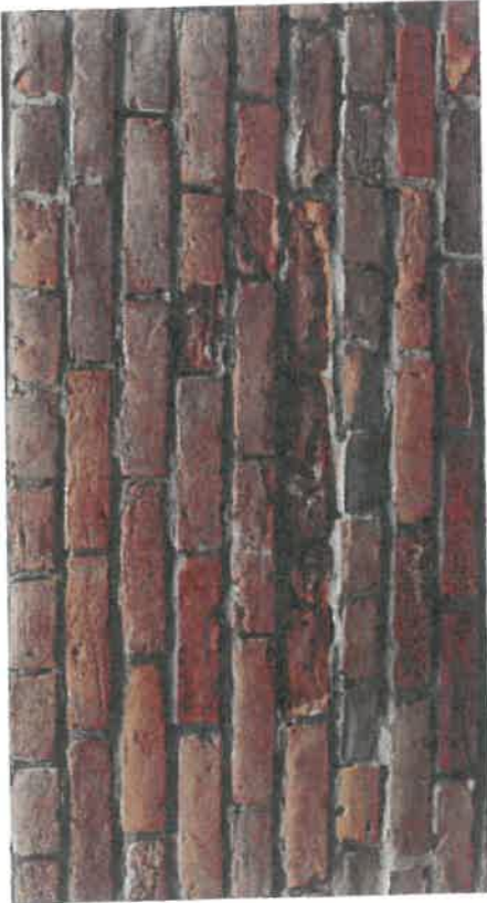
Example of deteriorated masonry and mortar. (STRATA)
