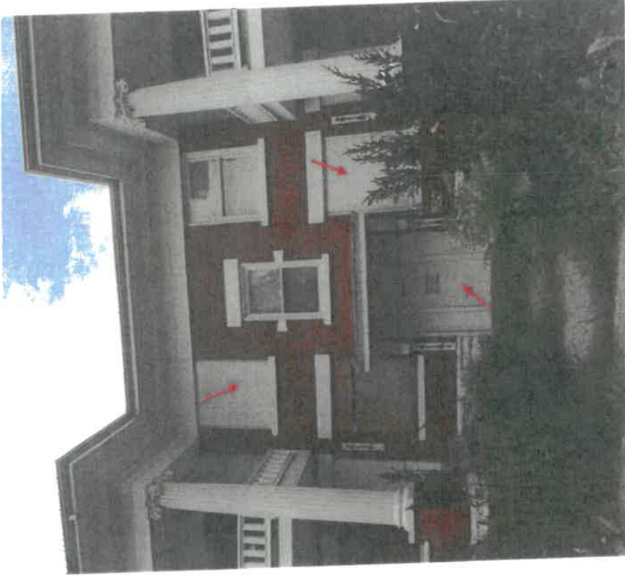
Example of temporary mothballing treatment. Note the mixture of good and poor mothball treatments. The door and a few of the windows (as noted with red arrows) are covered with painted, tight-fitting plywood, which will protect the building from vandalism and weather. The raw plywood has a gap between the pieces of plywood, which will allow water into the building, and two of the windows are not covered, which could be broken. (STRATA)
