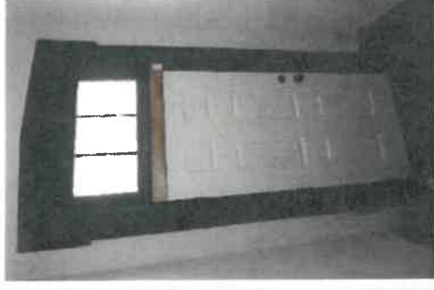
Example of inappropriate door replacement. The replacement door is too short and does not fit into the door opening. (STRATA)
