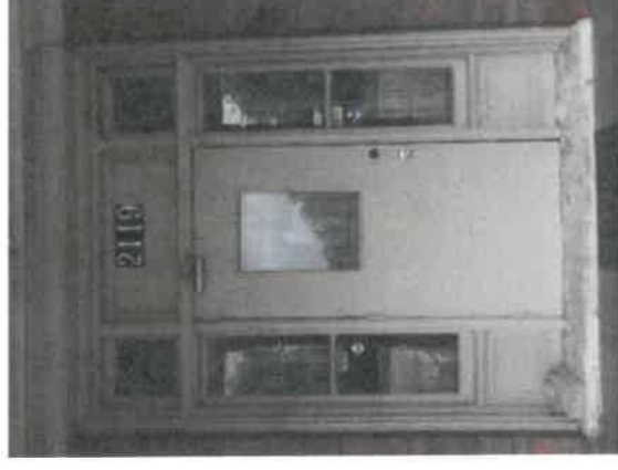
Example of an infilled transom. Infilling a transom is not permitted. (STRATA)
