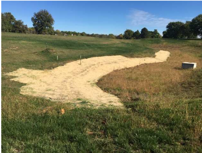
Photo Caption: Newly constructed detention basin with native grasses in bottom
