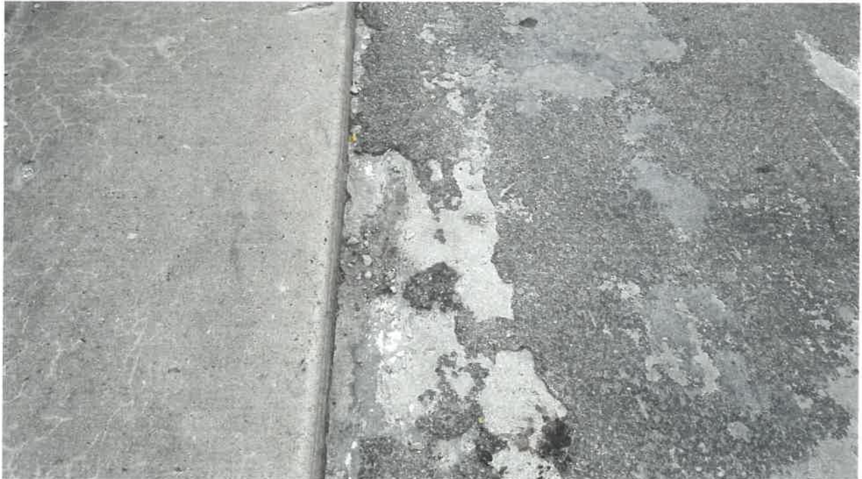
10. Asphalt Patching of Delaminated Sections
