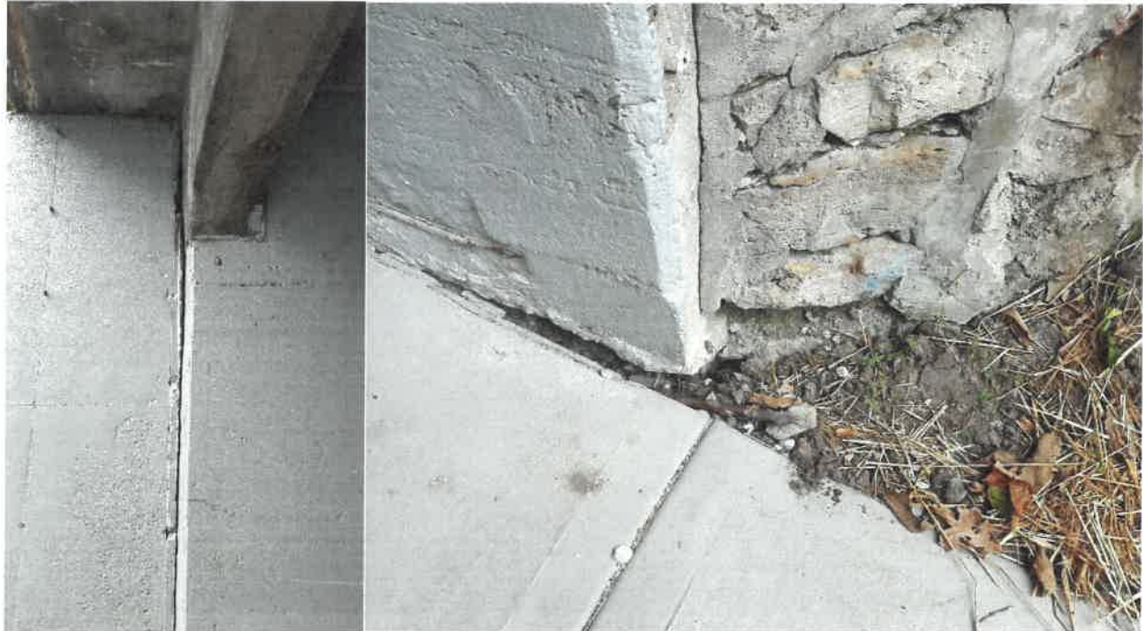
4. Evidence of Settlement (Northwest Corner, left; Northeast Corner, right).
