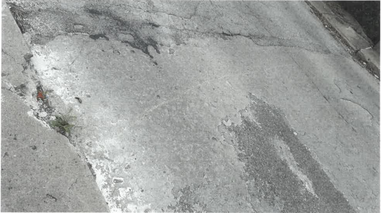
9. Indicated Section of Delamination from Non-Destructive Sound Test (North end of Road)
