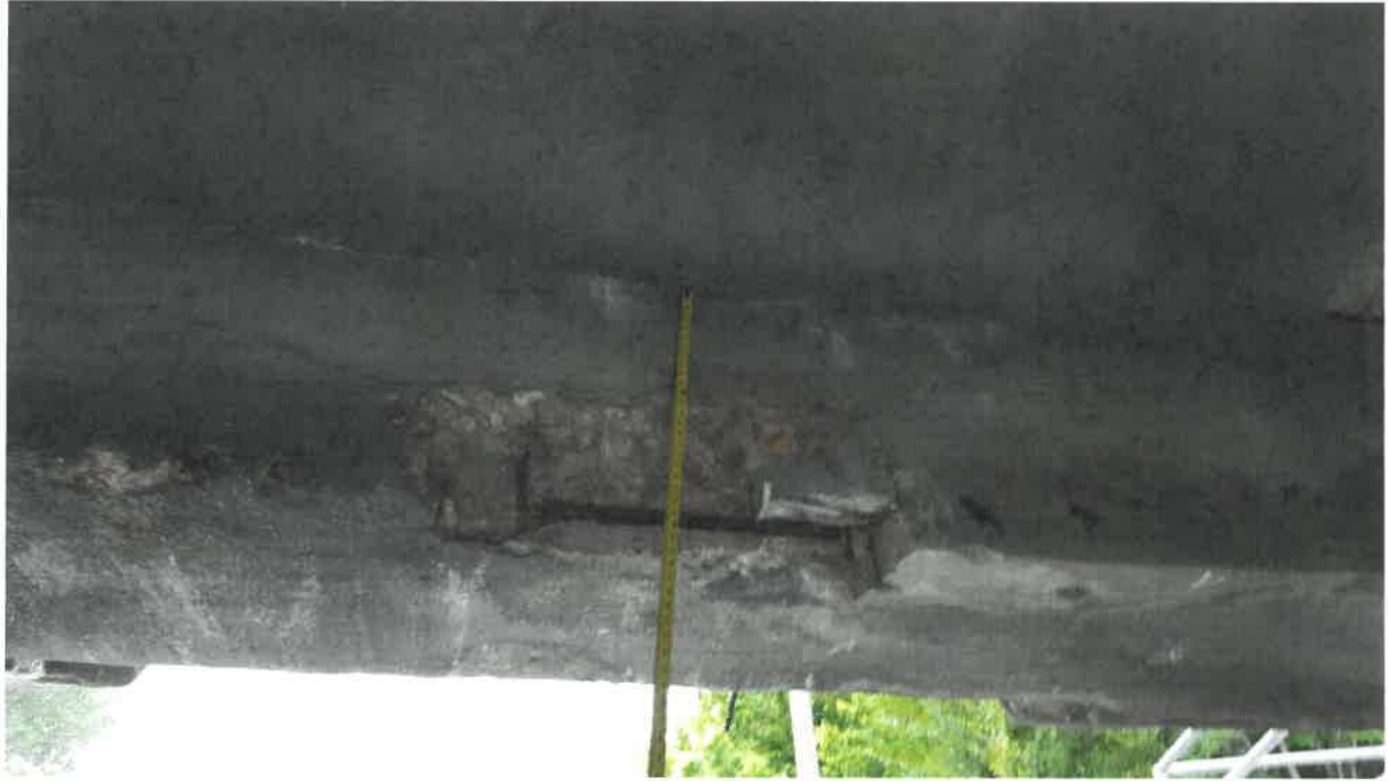
3. Exposed West Exterior Girder Reinforcement (Looking West).
